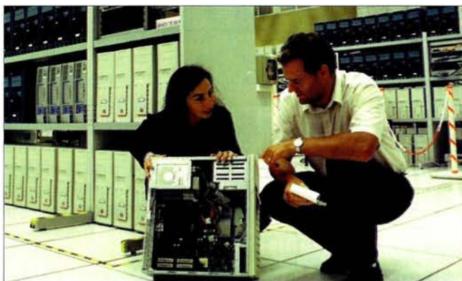
PC power: CERN's Computer Centre in 2001 has wall-to-wall PCs.
